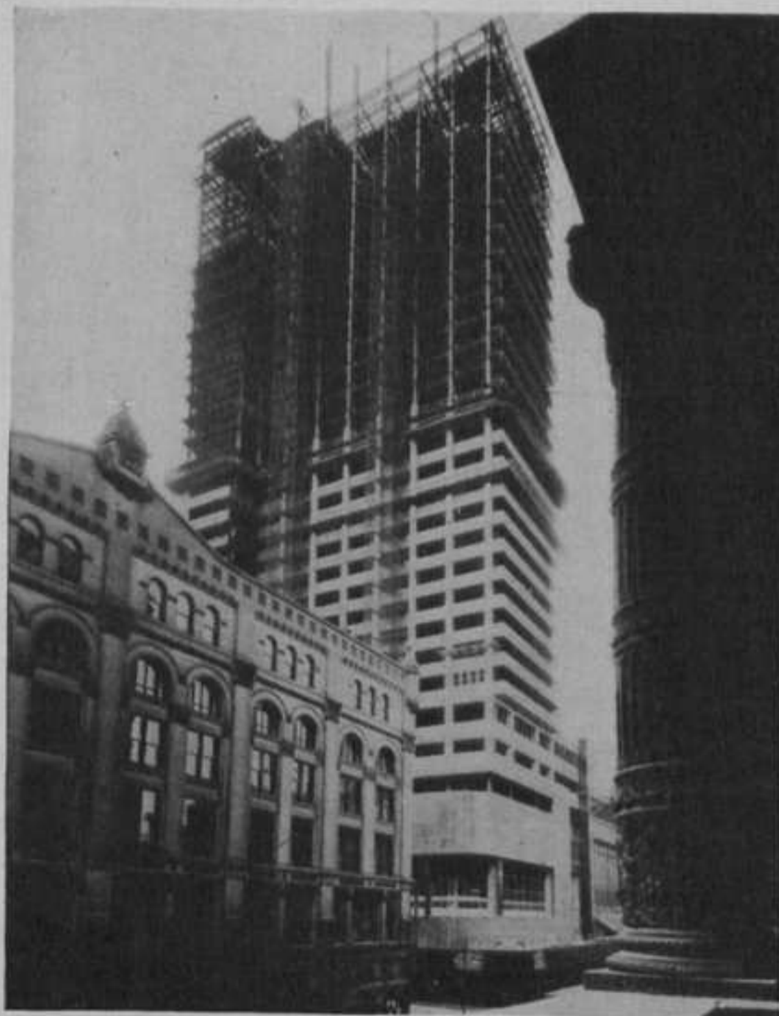
Fig. 1—Column pilasters in relief on the side faces and cantilever walls on the front face lend a new architectural note to the 33-story Savings Fund Society Building, tallest office structure in Philadelphia.
