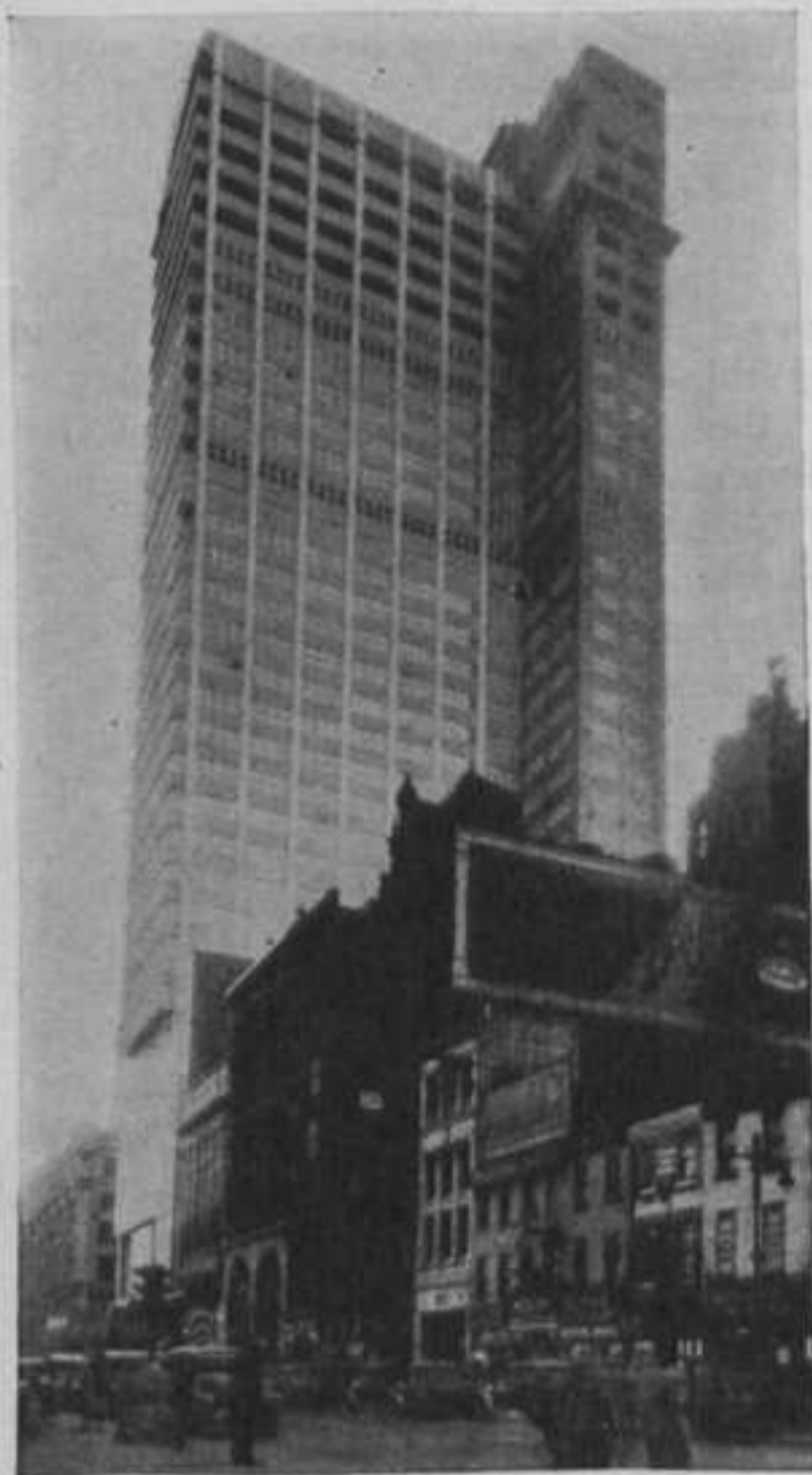
Fig. 4—In the completed building the rear wing, containing the service facilities and some offices, is inclosed in darker brick than the main-office portion in which the columns appear in relief except on the front facade, which is devoid of all columns.
