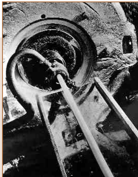
Extruder press forming rods of Pyralin cellulose nitrate plastic at the Arlington, New Jersey, plant of E. I. du Pont de Nemours & Co., mid 1930s. Pyralin was supplied to fabricators in the form of sheets, rods, and tubes.
