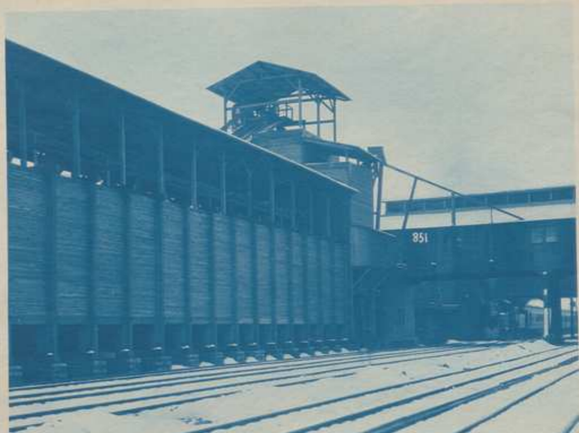
Side View of Cooling Station at Lyons, N.Y. - N.Y.C. & H.R.R.R. - showing Storage - Pocket and Cooling Bridge
