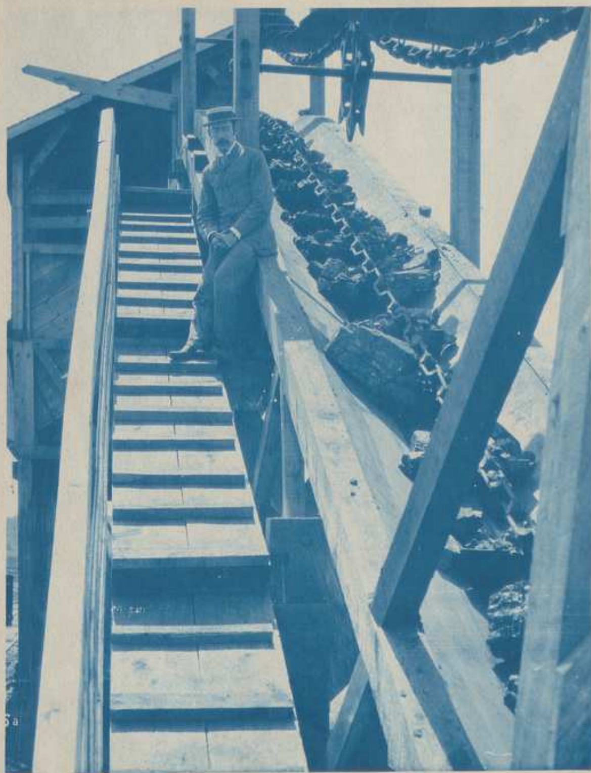
~ Inclined Conveyor handling Bituminous Coal - at - New Buffalo Coaling Station - C. & W. M. Ry. Co. ~
