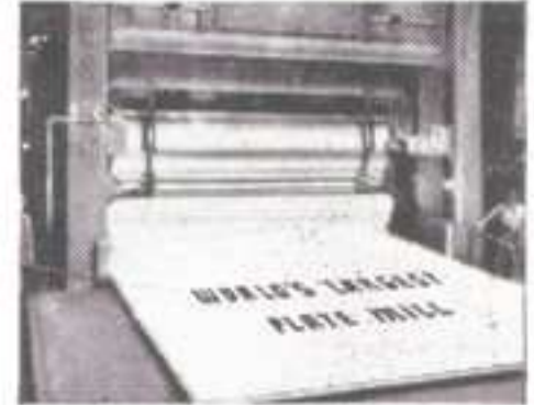
1940 THE WORLD'S LARGEST PLATE MILL
