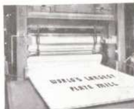
1940 THE WORLD'S LARGEST PLATE MILL
