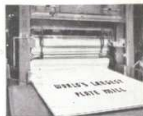
1940 THE WORLD'S LARGEST PLATE MILL
